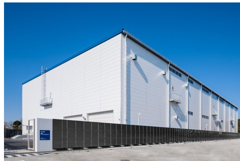
▲ Inzai Archives Center external view
