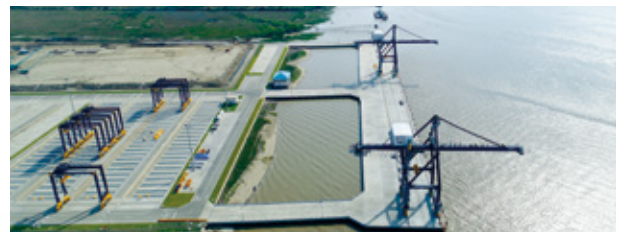
Myanmar Yangon Thilawa Port Expansion Project
