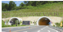
Vietnam Hai Van Tunnel Construction Project
