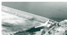
Vietnam Da Nhim Hydropower Project
