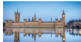
United Kingdom Palace of Westminster Restoration and Renewal Project
