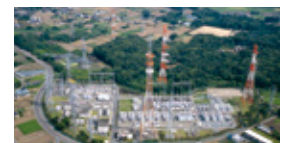
Japan Shin Sakado Substation High-capacity transmission and substation facilities
