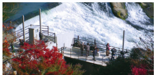
Japan Shinsogi Power Plant
