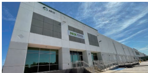
New warehouse in San Antonio, Texas
