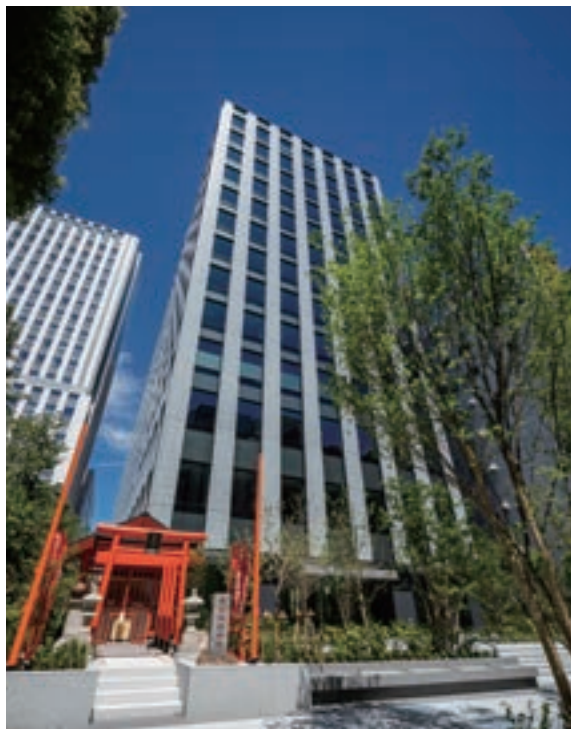
Exterior of NX Group Building
