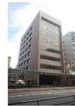
Hachioji-shi, income-generating office
