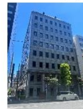
Chuo-ku, income-generating office
