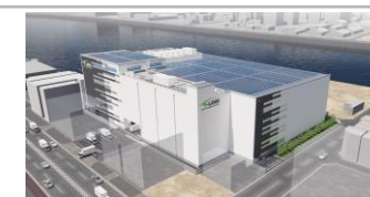
T-LOGI Osaka Bentencho (Under Development)
