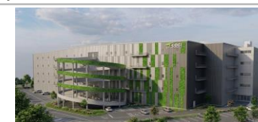
T-LOGI Kashiwa・Noda (Under Development)
