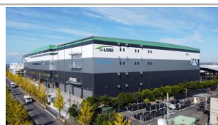
T-LOGI Kuki (Completed)
