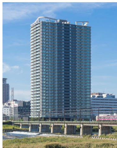
▲ Brillia Tower Seiseki Sakuragaoka BLOOMING RESIDENCE (adopted as the Tokyo Metropolitan area's first ultra-high-rise ZEH-M pilot project)
