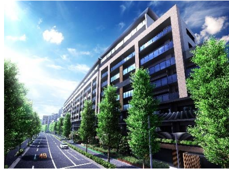
▲ Livio City Bunkyo Koishikawa (Total units: 532; Units to be posted: 79)
