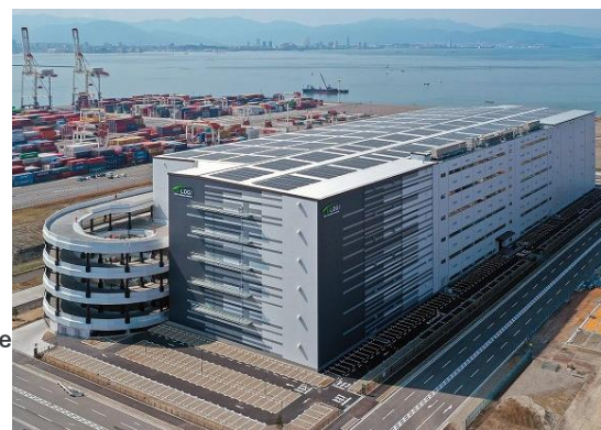
▲ T-LOGI Fukuoka Island City (Completed in 2024)
