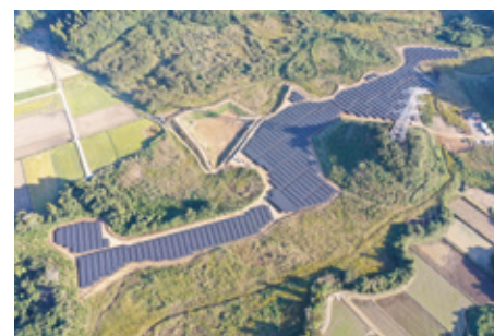
Solar power plant in Chiba Prefecture
