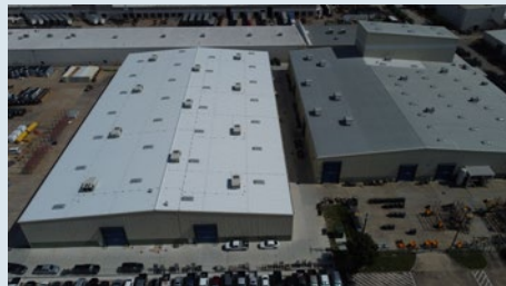
New factory under construction
