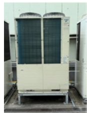
Upgrade to EHPs (Kyoto Plant)
