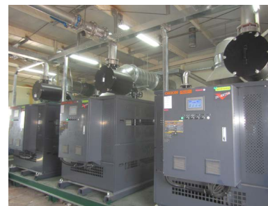
Air-cooled vacuum pump
