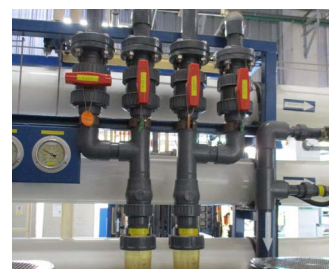
Piping for sending recycled water to the cooling tower
