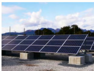
Hongo Photovoltaic Power Plant
