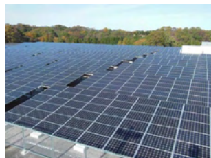
Elna Shirakawa Photovoltaic Power Plant
