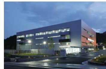
The energy-efficient Himeji Parts Center.
