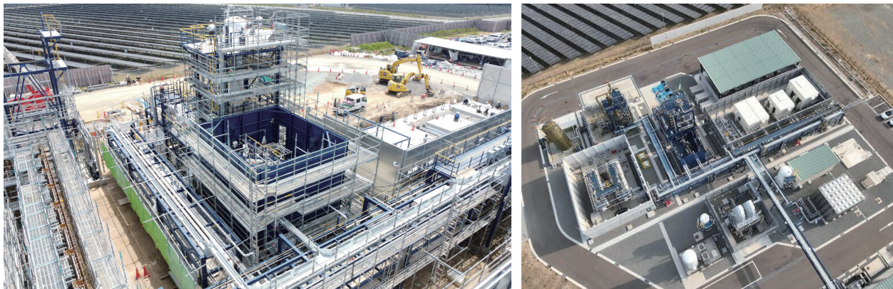
Green ammonia production demonstration plant Left: Construction in progress Right: Plant overview (supplied by JGC)
