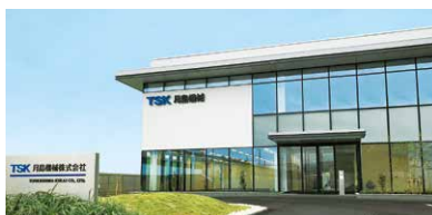
R&D Center, outside view
