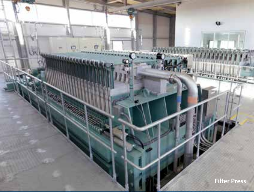
Sewage Sludge Dewatering and Drying system (demonstrated in B-DASH national project)
