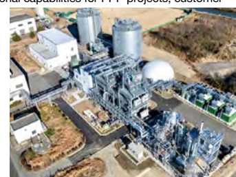
Iwaki sewage sludge recycling project (PFI project)
