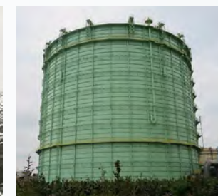
Gas holder Highly earthquake-resistant dry sealed gas holder
