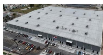
Automatic door plant in Mexico
