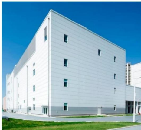
Completed Phase 2 manufacturing building
