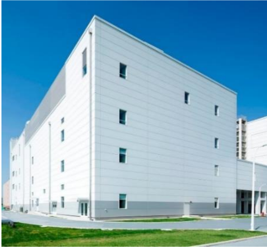
Completed Phase 2 manufacturing building
