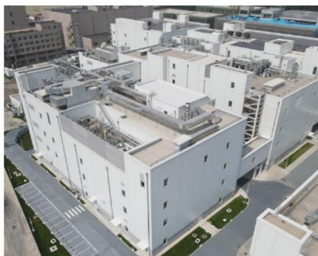
Newly-constructed Tianjin Plant
