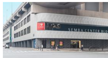
Osaka Semba Center Building
