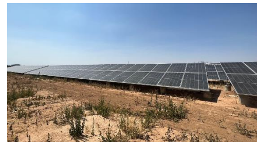
Solar power plant in Sabha, Mafrq (Jordan)
