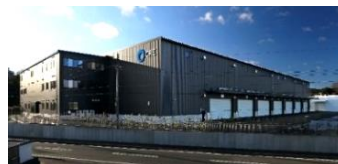
LogiSquare Kakegawa (Shizuoka Prefecture) total floor area: 14,236sqm
