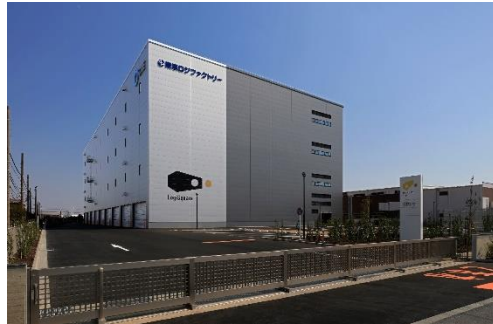
LogiSquare Atsugi II (Kanagawa Prefecture) total floor area:18,422sqm
