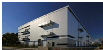
LogiSquare Itami (Hyogo Prefecture) total floor area: 29,978sqm
