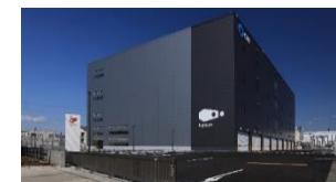
LogiSquare Atsugi I (Kanagawa Prefecture) total floor area: 18,236sqm
