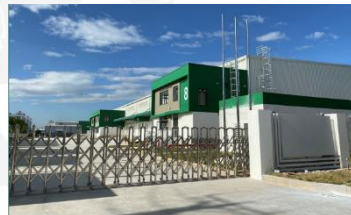
Sembcorp Logistics Park (Quang Ngai) Park B
