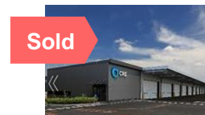
LogiSquare Narita (Chiba Prefecture) total floor area: 18,022sqm
