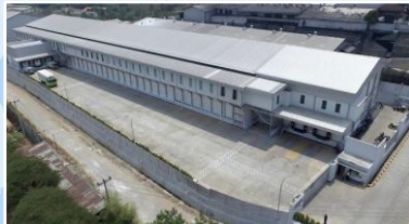
Cella Gemilang Logistik Warehouse (Narogong)
