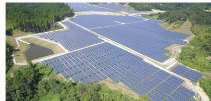
ReENE Chonan Solar Power Plant (Chiba) Rated capacity: 24 MW
