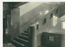
Restoration of a marble staircase with strong historical value
