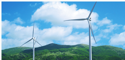
ReENE Matsumae Wind Power Plant (Hokkaido) Rated capacity: 41 MW
