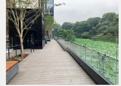
Terrace along moat
