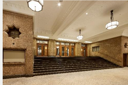
Entrance hall utilizing marble from the original construction
