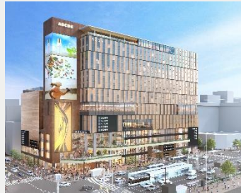
COCONO SUSUKINO (Sapporo Susukino Ekimae Complex Redevelopment Project) Sapporo, Hokkaido Hotel/Commercial/Cinema, etc. Floor space: 53 Scheduled to open in November in 2023
