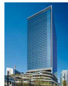
TOKYO PORTCITY TAKESHIBA Office tower Minato-ku, Tokyo
