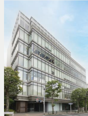
Meguro Tokyu Building
