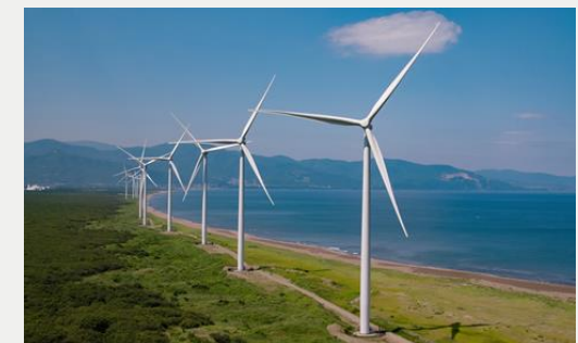
ReENE Zenibako in Hokkaido Wind power plant : 34MW
