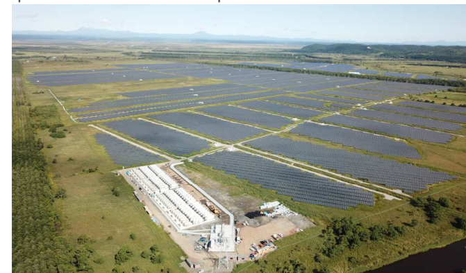
Suzuran Kushiro-cho Solar Power Plant : 92MW (Operation started in February 2020)
