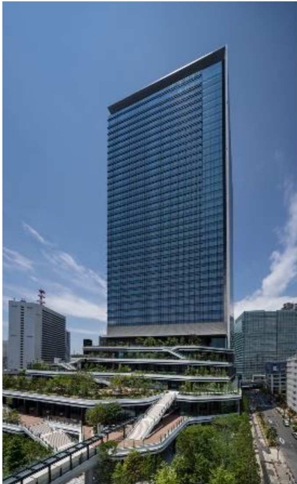
Office tower Office/Commercial Floor space : about 182 thousand m 2 Complete : May, 2020
