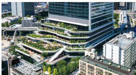
TOKYO PORTCITY TAKESHIBA (Completion: May 2020)
