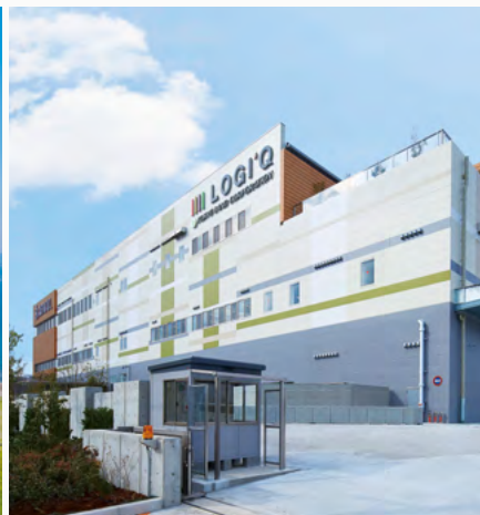
LOGI'Q Miyoshi (Completion: January 2020)
