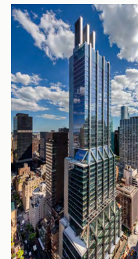
425 Park Avenue (Completion: January 2021)
