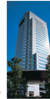
1993 Setagaya Business Square Tokyu Group's first super-high-rise office building
