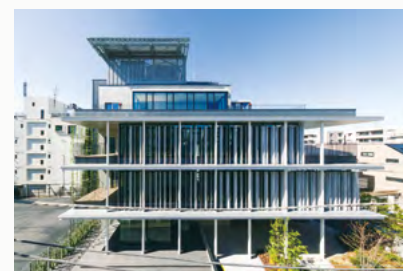
Tokyu Community Technology Training Center NOTIA (with a Nearly ZEB certification)
