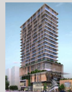
Chayamachi B-2 Block Urban Redevelopment Project Osaka Commercial, etc.
