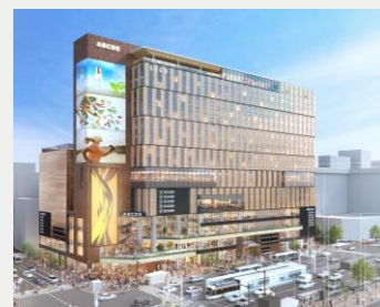
Sapporo Susukino Ekimae Complex Redevelopment Project** Sapporo Hotel/Commercial/Cinema, etc. Floor space : 53 Open : FY2023 (Plan)
