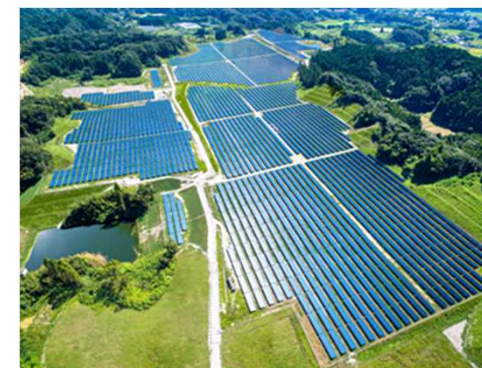
ReENE Chonan Solar Power Plant(Chiba prefecture) : 24MW (Operation started in July 2020)
