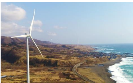
ReENE Matsumae Wind Power Plant
