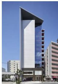
Namba Motomachi 1-chome Place Osaka Hotel Floor space : 5
