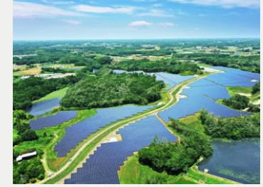
ReENE Namegata Solar Power Plant (Ibaraki) Rated capacity: 28MW (Operation started in 2020)
