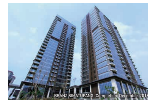
BRANZ SIMATUPANG (Completion: December 2018)
