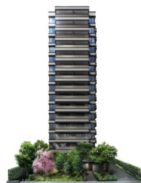
BRANZ Rokuban-cho (To be completed in February 2019)
