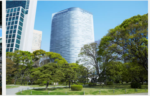
Dentsu Headquarters Building
