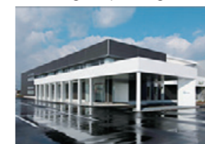
Yonago Operations Center (Yonago City, Tottori Prefecture)
