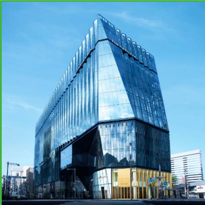
Tokyu Plaza Ginza Usage: Commercial Floor Space: approx. 51,000m 2 Open: Mar-31, 2016
