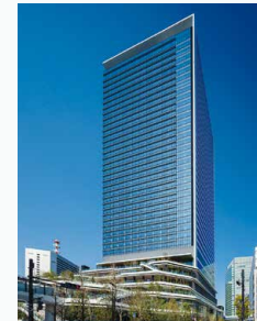
TOKYO PORTCITY TAKESHIBA Office tower Minato-ku, Tokyo
