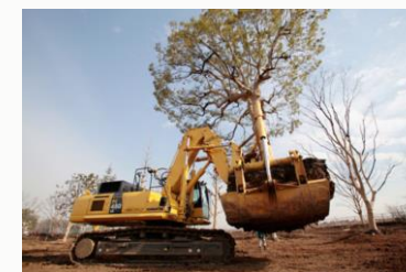
Transplanting work using a TPM machine
