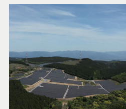
ReENE Ebino Solar Power Plant
