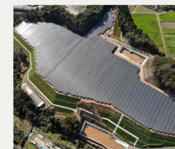
ReENE Izumi Solar Power Plant
