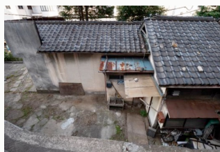
The previous street layout. Non-fire-resistant buildings and narrow roads that fire trucks could not access
