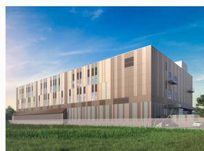
100% renewable energy-powered data center (Ishikari-shi, Hokkaido)
