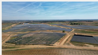
Valdecarretas Solar Power Plant* (Spain)
