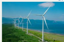
ReENE (Wind power generation facilities)
