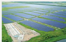
ReENE (Solar power generation facilities)
