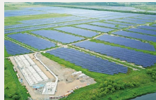
ReENE (Solar power generation facilities)
