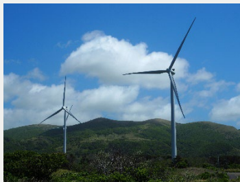
ReENE Matsumae Wind Power Plant (Hokkaido) Rated capacity: 41MW (Operation started in FY2019)
