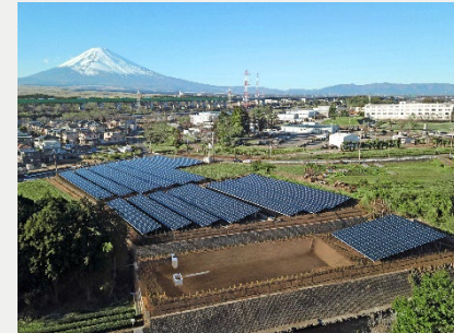
ReENE Shizuoka Kamiyama Solar Power Plant providing electricity directly to our own facilities
