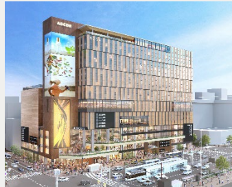
COCONO SUSUKINO (Sapporo Susukino Ekimae Complex Redevelopment Project) Sapporo, Hokkaido Hotel/Commercial/Cinema, etc. Floor space : 53 Scheduled to open in Autumn in 2023
