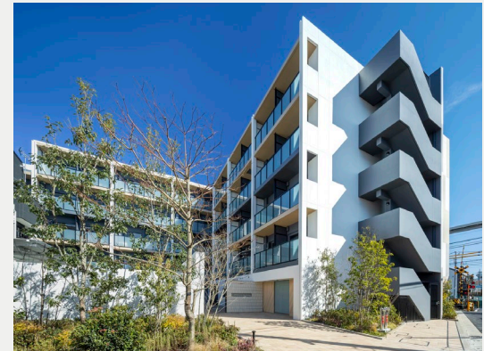
CAMPUS VILLAGE Chitose Karasuyama (Completed in March 2023; total student residence units: 182)
