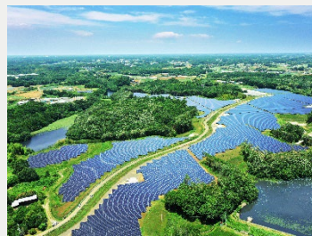
ReENE Namegata Solar Power Plant (Ibaraki) Rated capacity: 28MW (Operation started in FY2020)
